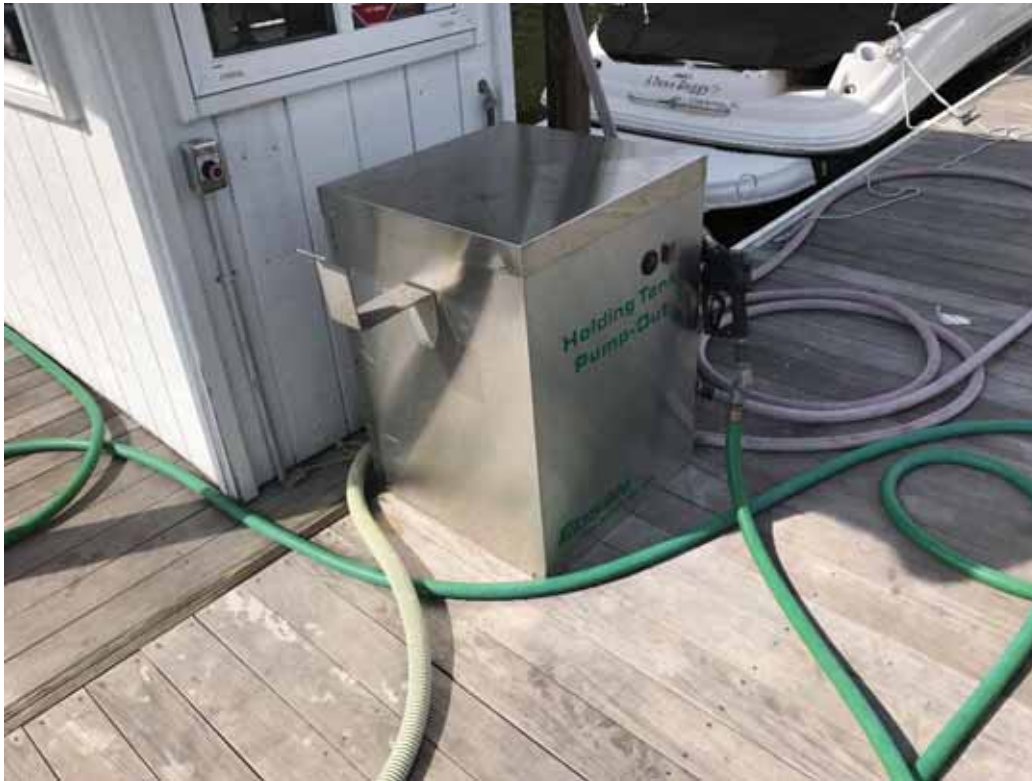
Photograph 7: View of the holding tank/pump-out at the fuel dock at the marina.
